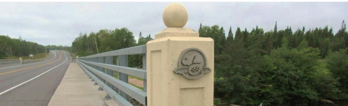
Bridge on the Trans-Canada Highway in Terra Nova National Park, 2019
