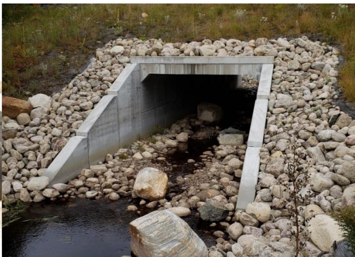
Image: A culvert before and after major rehabilitation in La Mauricie National Park, 2019. Among other features, the culvert was made deeper to help aquatic life cross through.
