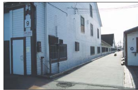
West exterior wall of Cannery
