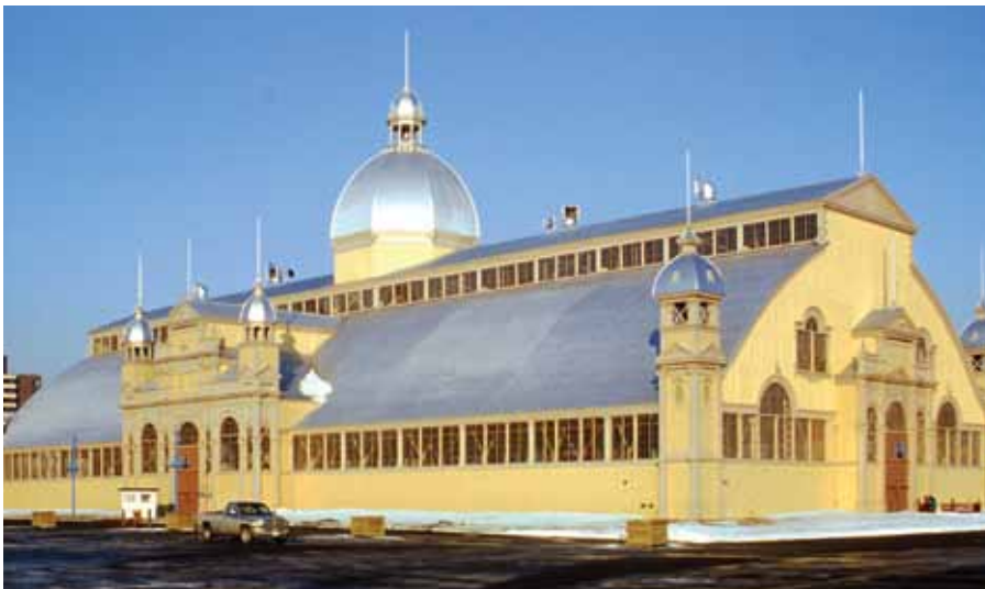
The windows of the Aberdeen Pavilion in Ottawa, a building that is valued as an example of a large-scale exhibition structure from the 19 th century, include monitor windows at the top of the curved roof structure to provide daylight to the wide open space from above. Preservation of the character-defining wood windows involved scraping, sanding, re-puttying and repainting. While some replacement in kind was undertaken, almost all the original windows were retained, including the glass. Wholesale replacement of window units is not an appropriate Preservation treatment.
