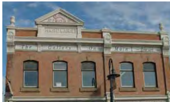
Under certain circumstances, substitute materials may be appropriate. As part of a Rehabilitation project, new finials were designed based on original remains. The originals were fabricated of wafer-thin galvanized metal soldered together. The substitute material used in the new design was plate aluminum.
