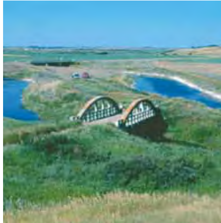
The Eagle Creek Cement Bridge in Saskatchewan is a good example of the nearly 90 reinforced concrete bowstring bridges that were constructed during the 1920s and 1930s as part of a comprehensive road building program in southern Saskatchewan. The graceful bowstring arches of these bridges, which blended functional engineering technology with aesthetically pleasing design, are character-defining elements. Repair or replacement of any parts of the bowstring arches should carefully designed for compatibility, matching the original form, materials and detailing of the arches.
