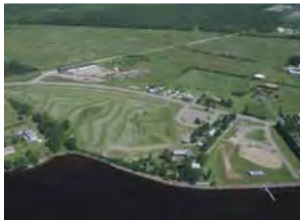
The Bonar Law House is a 9 hectare property along the north side of the Richibucto River in the Village of Rexton, NB. This complex contains a simple 19 th century wood farm house facing the river and a barn and wagon shed. Board fencing connects the buildings to form an enclosed courtyard. New community facilities are being implemented to increase community use while maintaining the site's original spatial organization.
