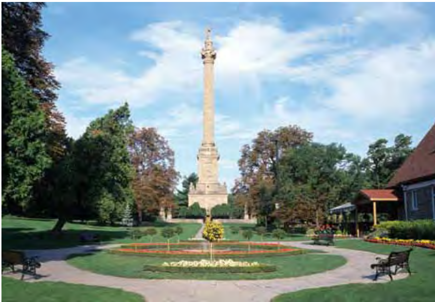
Many stone masonry monuments, such as the Brock Monument in Queenston, ON, are historic places. A monument does not face many of the challenges of historic buildings or engineering works. Its purpose and use are the same today as when it was built. A monument is expected to remain constant and unchanged despite time, deterioration and weathering. Continuous maintenance and repairs are required and interventions or major repairs must be carefully considered to evaluate their potential impact on each part of the monument.
