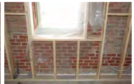
Left: Interior of west (rear) wall of north retail bay, showing as-found condition of load-bearing masonry after removal of the lath and plaster interior finishes for inspection purposes. Uncontrolled runoff from the roof had saturated the wall, washed out the mortar, and caused localized collapse around the window opening.
