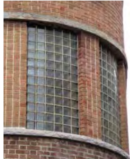
Glass block has been manufactured in many different shapes, sizes, patterns and opacities. All these features should be considered when seeking a replacement block. Searching architectural salvage yards and contacting manufacturers may locate compatible replacements.
