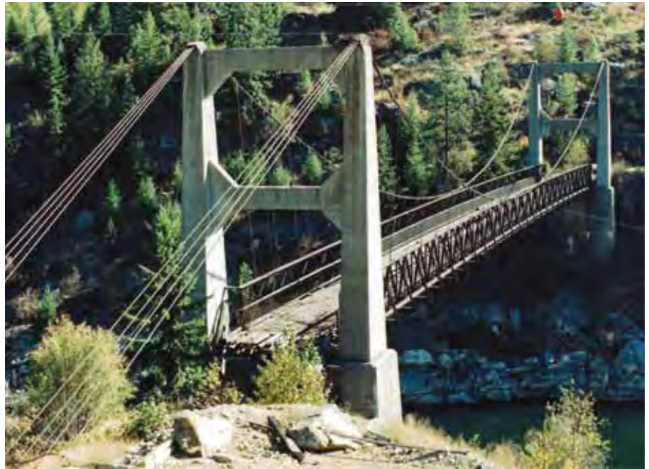
The Doukhobor Suspension bridge, near Castlegar, BC, is an example of a civil engineering work with significant cultural symbolic value. Erected by members of the Doukhobor community, its construction represents a major achievement for a pioneer community and demonstrates the considerable capabilities of a people acting communally.
