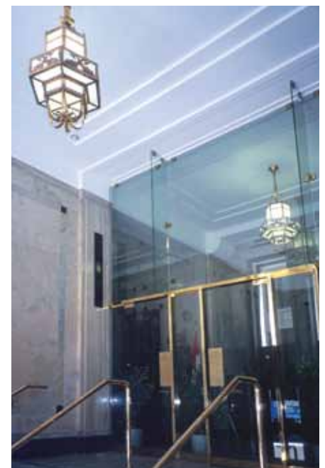
When adding any new features to meet functional requirements, adjacent character-defining elements should be conserved. A new glass wall in the Dominion Public Building in Halifax was carefully designed to complement the quality of the lobby's materials and finishes, and installed to avoid damaging the adjacent character-defining plasterwork and stone wainscoting.
