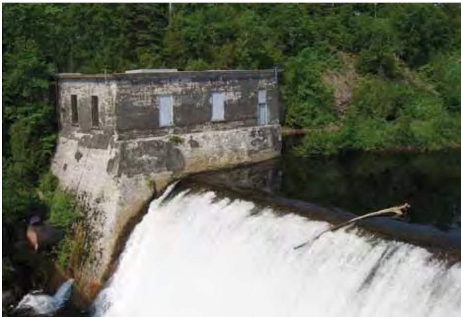
Remains of hydroelectric installations.
