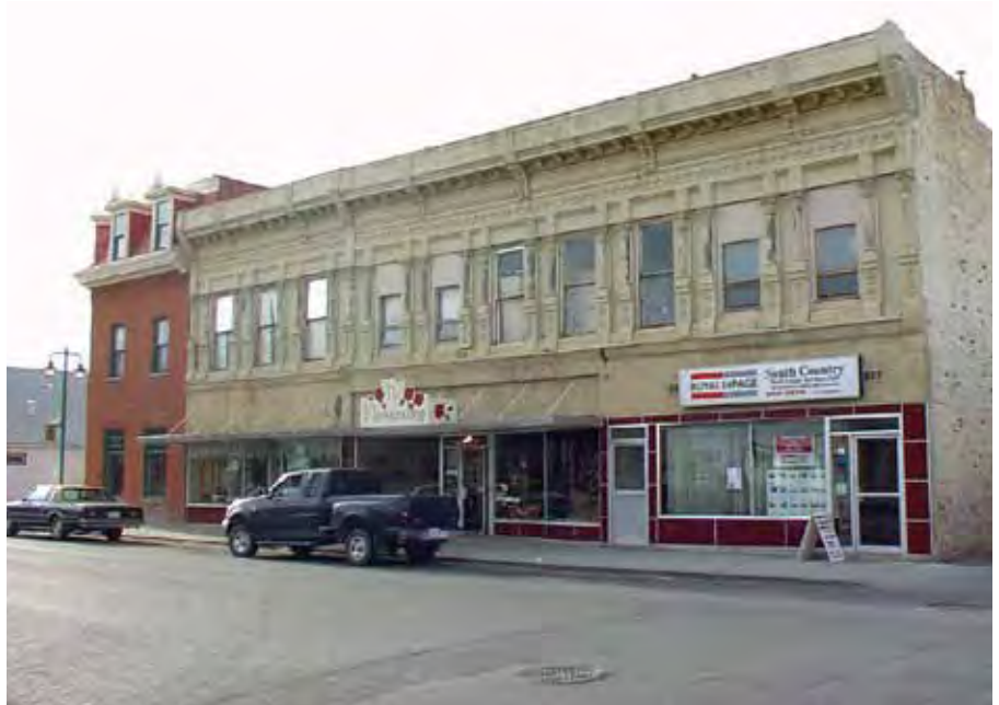
Before rehabilitation: east façade, looking southwest.
