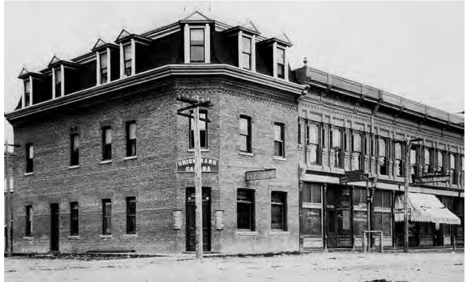
1906 photograph of Grier Block (at right) from southeast.
