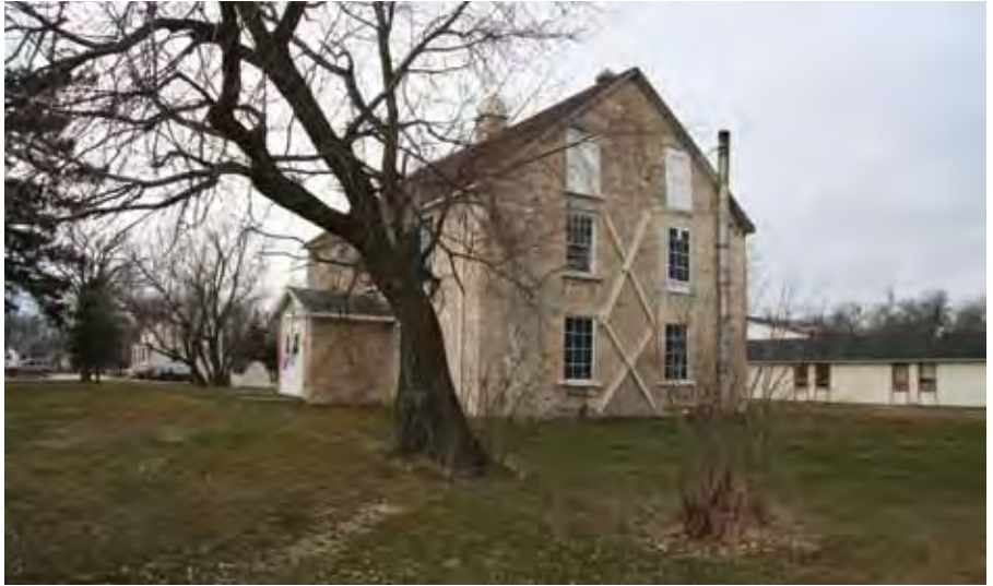
It is important to adapt interim stabilization interventions to the anticipated lifespan of the intervention and make it as reversible as possible. Temporary steel cross bracing supports an exterior wall at St. Peter's Dynevor Anglican Church Rectory in Selkirk MB.
