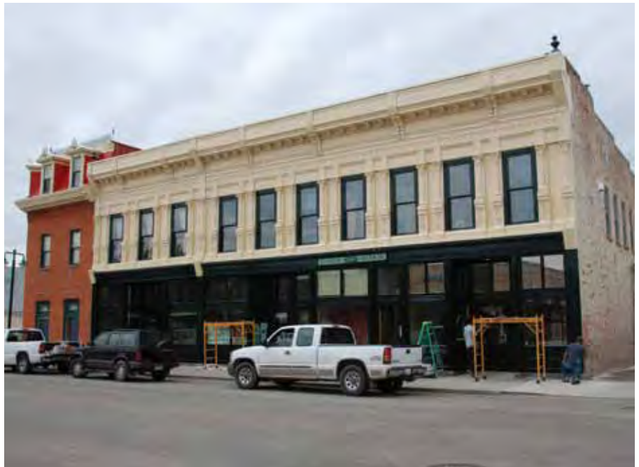
East façade after restoration of storefronts and preservation of pressed metal façade. Maintenance (repainting) in progress.
