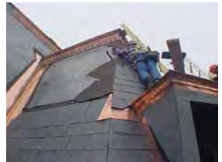
The Rehabilitation of the Truro Post Office, in Truro, NS included restoring its distinctive slate roof. In Rehabilitation, the replacement of missing historic features with a replica based on physical and documentary evidence, as in this project, is acceptable, as is a new design that is compatible with the heritage value of the historic place.
