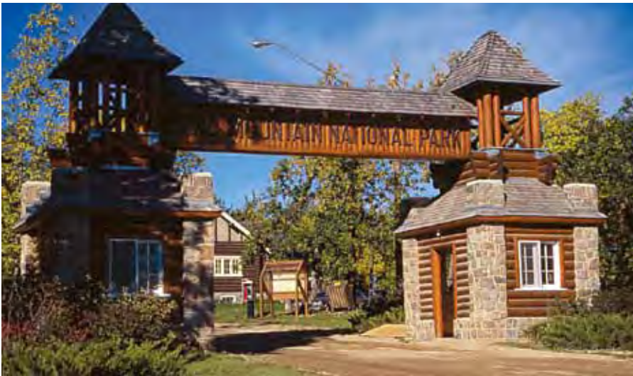
The East Gate Entrance Building at Manitoba's Riding Mountain National Park is a character-defining element of this cultural landscape that needs to be protected.
