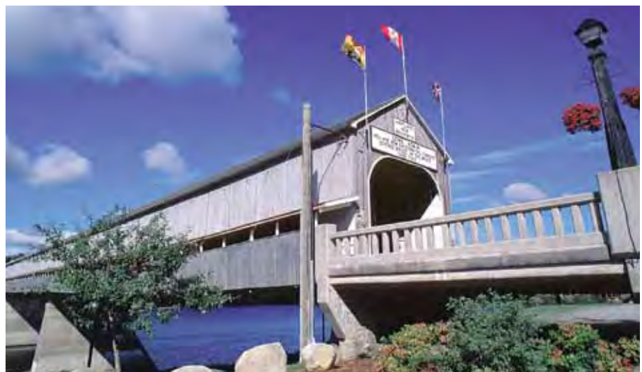
The Hartland Covered Bridge, crossing the St. John River at Hartland, NB, is the world's longest covered bridge. It is significant for its structural qualities, contributions to transportation and as a symbol of the heritage of covered bridges in New Brunswick. The present bridge is a standard covered bridge structure composed of a Howe truss superstructure enclosed with vertical unpainted weatherboard siding. When the New Brunswick Department of Transportation recently rehabilitated the bridge by installing a fire suppression system, care was taken to ensure that this new system was barely visible in the upper structural system.
