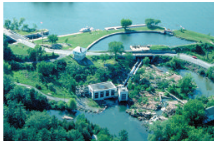
The slackwater system often entailed the construction of a system of dams, as at Kingston Mills.
