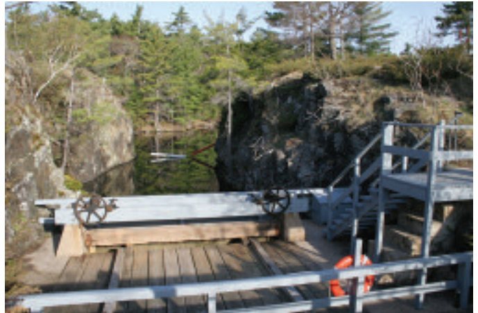
The Jones Falls weir is part of the complex system of dams at this lockstation.
