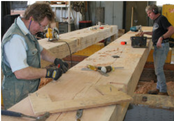
Gates have a life span of up to twenty-five years. New gates are made by Parks Canada Agency staff, following the design of the originals.
