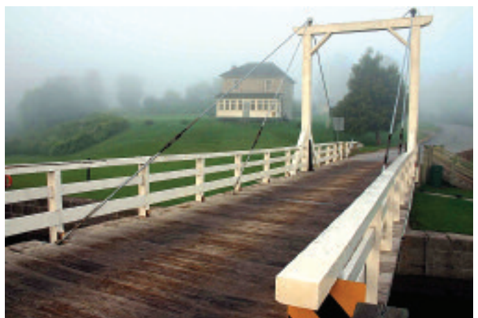
Authentic designs were used to construct the king post swing bridges found today at some lockstations.
