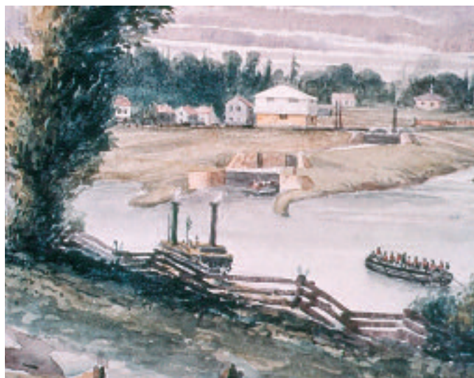
13 The blockhouse built to protect the locks at Merrickville.
