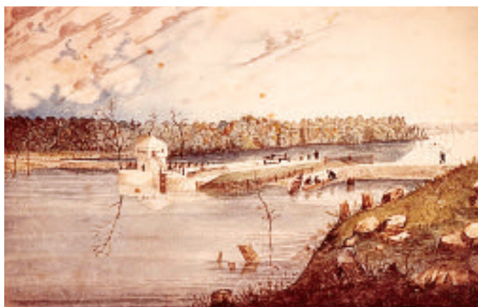
08 The lock, weir and 400-m-long earth embankment dam at The Narrows created a slackwater section allowing navigation to Newboro Lockstation.
