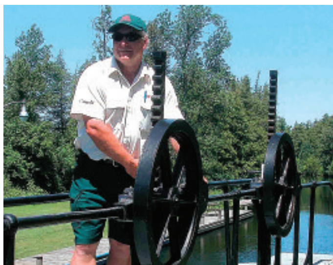
Lock gates and sluice valves are still operated using hand-powered winches.
