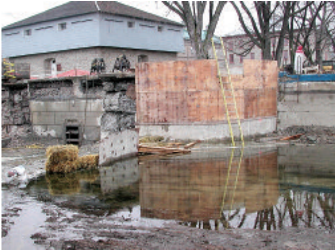
The climate of the area requires regular monitoring and repair of the limestone structures of the canal.
