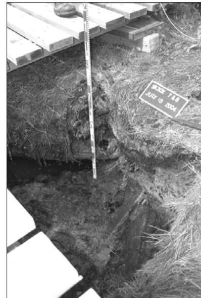
Thermokarst sinkhole in courtyard of the Depot, likely a result of drainage problems. (L. Dueck)
