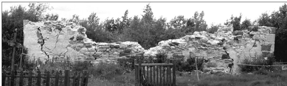
The deteriorating masonry of the Powder Magazine. (B. Lucki)
