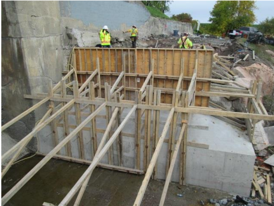
Kingston Mills Fixed Bridge Rehabilitation
