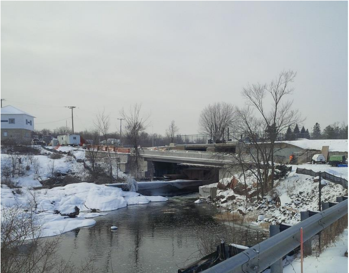
Kingston Mills Fixed Bridge Replacement
