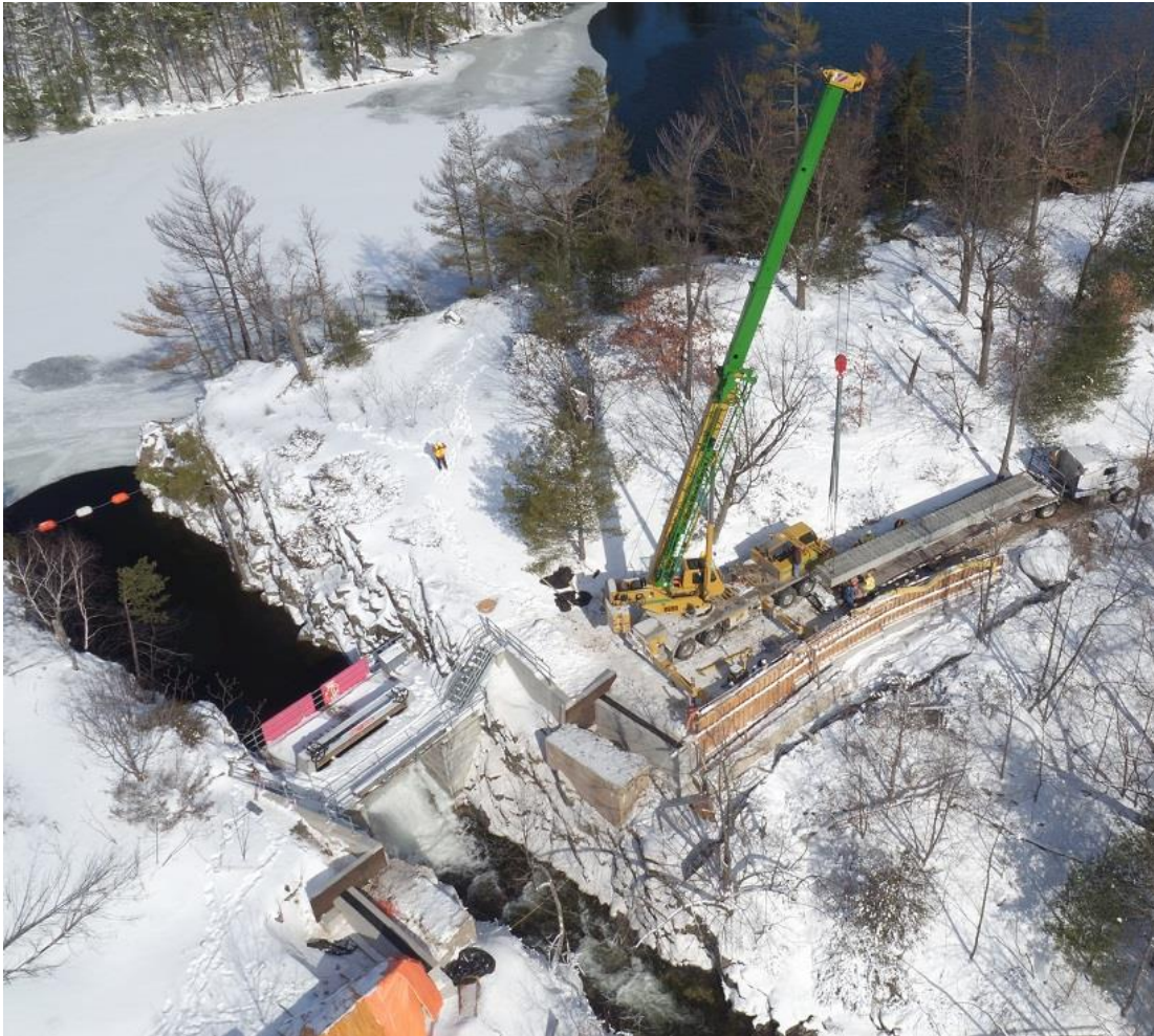
Girder installation at Jones Falls Concrete Bridge
