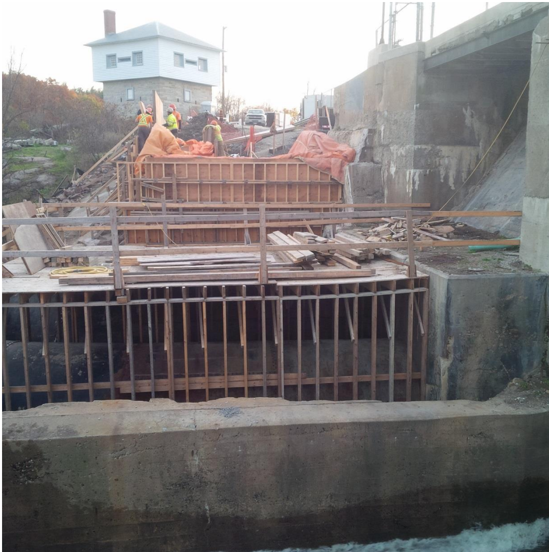
Kingston Mills Fixed Bridge Rehabilitation
