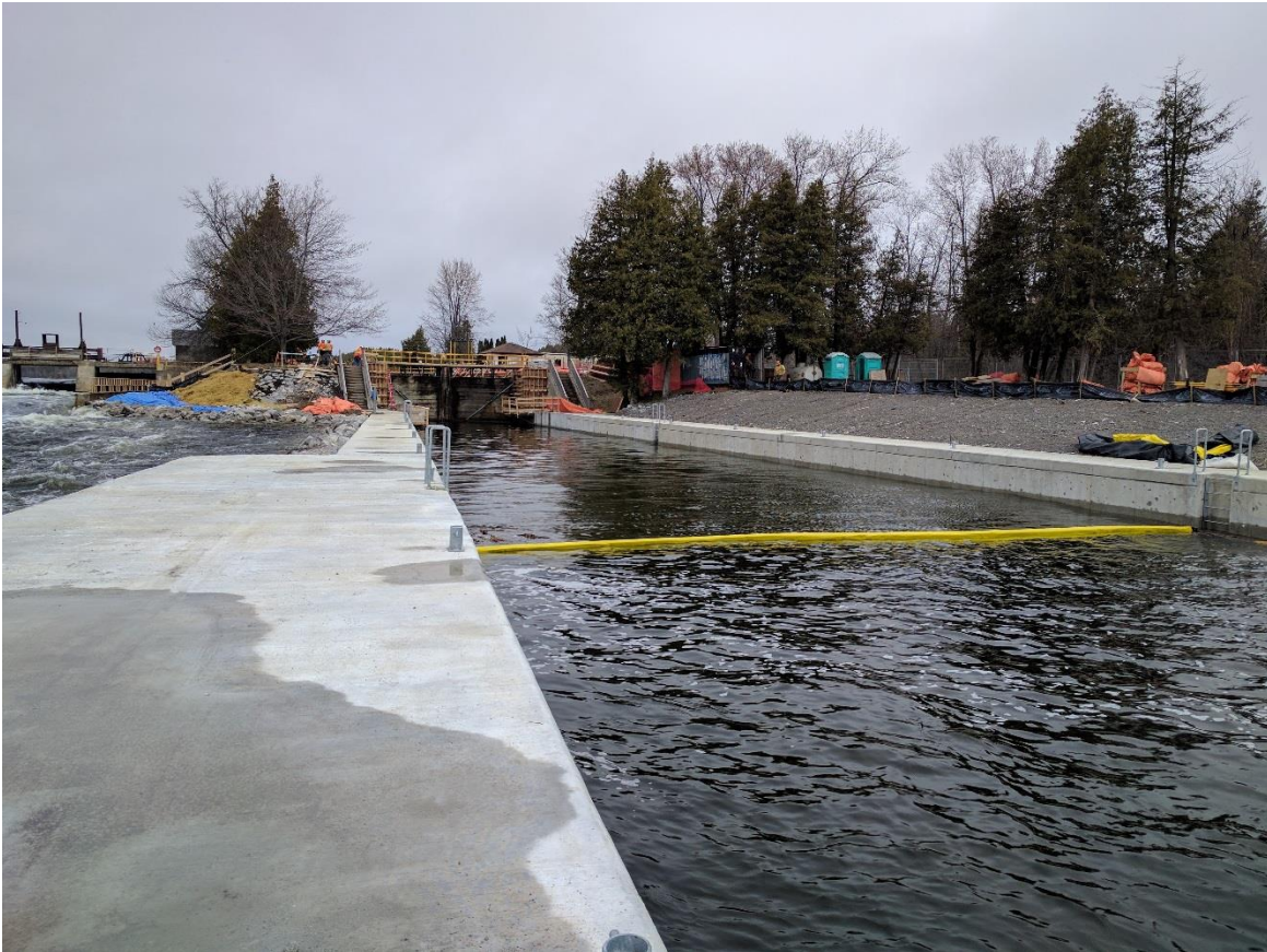
Sawer Creek Lock 25 Repairs
