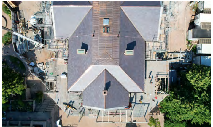
A drone image of the completed roof work.
