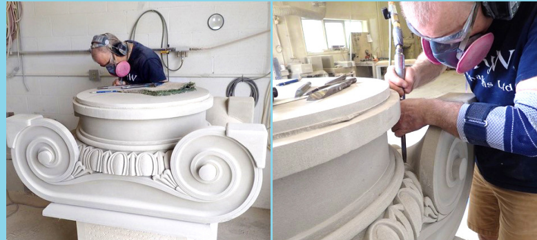
A skilled craftsperson applies the final decorations on the Ionic Capital that will be installed on the south west column of the south portico. Submitted by Trevor Gillingwater, stone conservator consultant for the Province House National Historic Site conservation project
