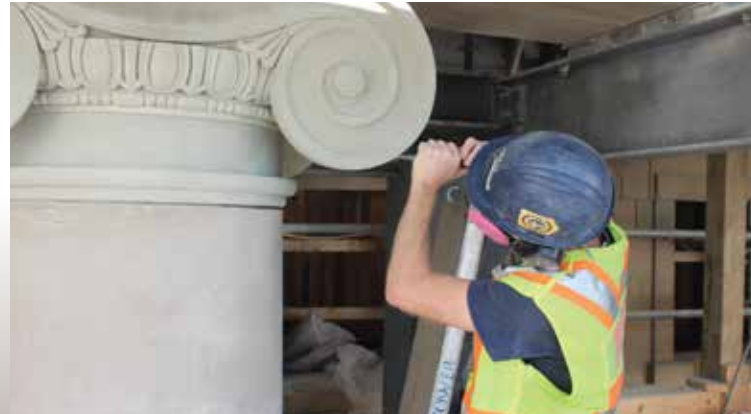
Robert Morrison carving the volutes (the scroll-like embellishment on the ionic capital stone) at Province House National Historic Site.
