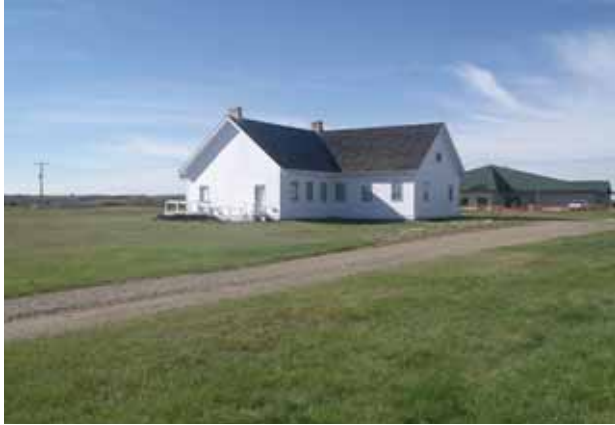
Barracks No. 5 with the Visitor Centre behind. (Parks Canada)
