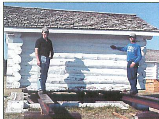
Repairing the Remount Ranch buildings at Fort Walsh NHSC. (Parks Canada)
