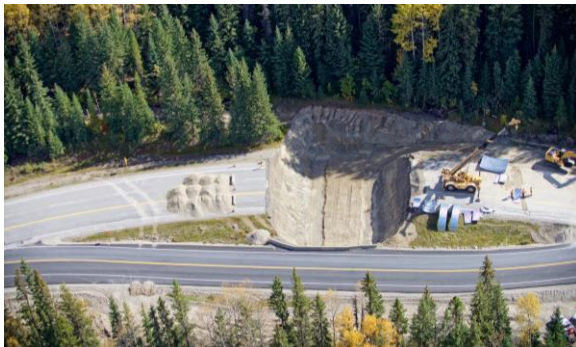
One of six new underpasses under construction in the fall 2015.
