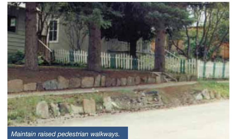
Protect existing stone walls.
