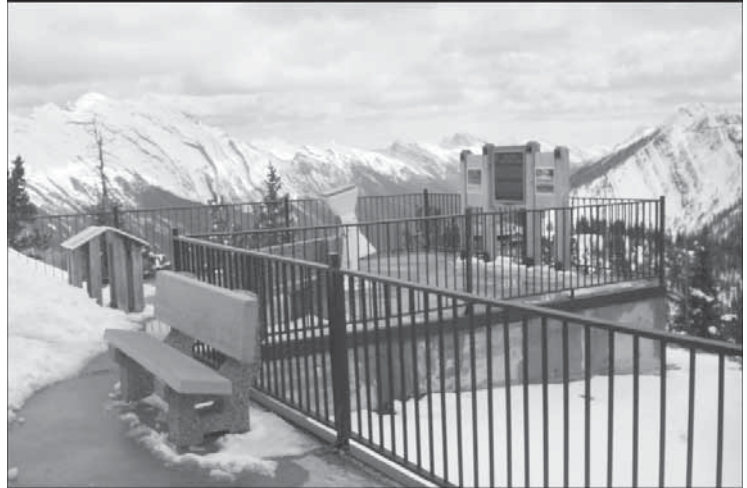
Surviving concrete foundation of the Sulphur Mountain Cosmic Ray Station.
