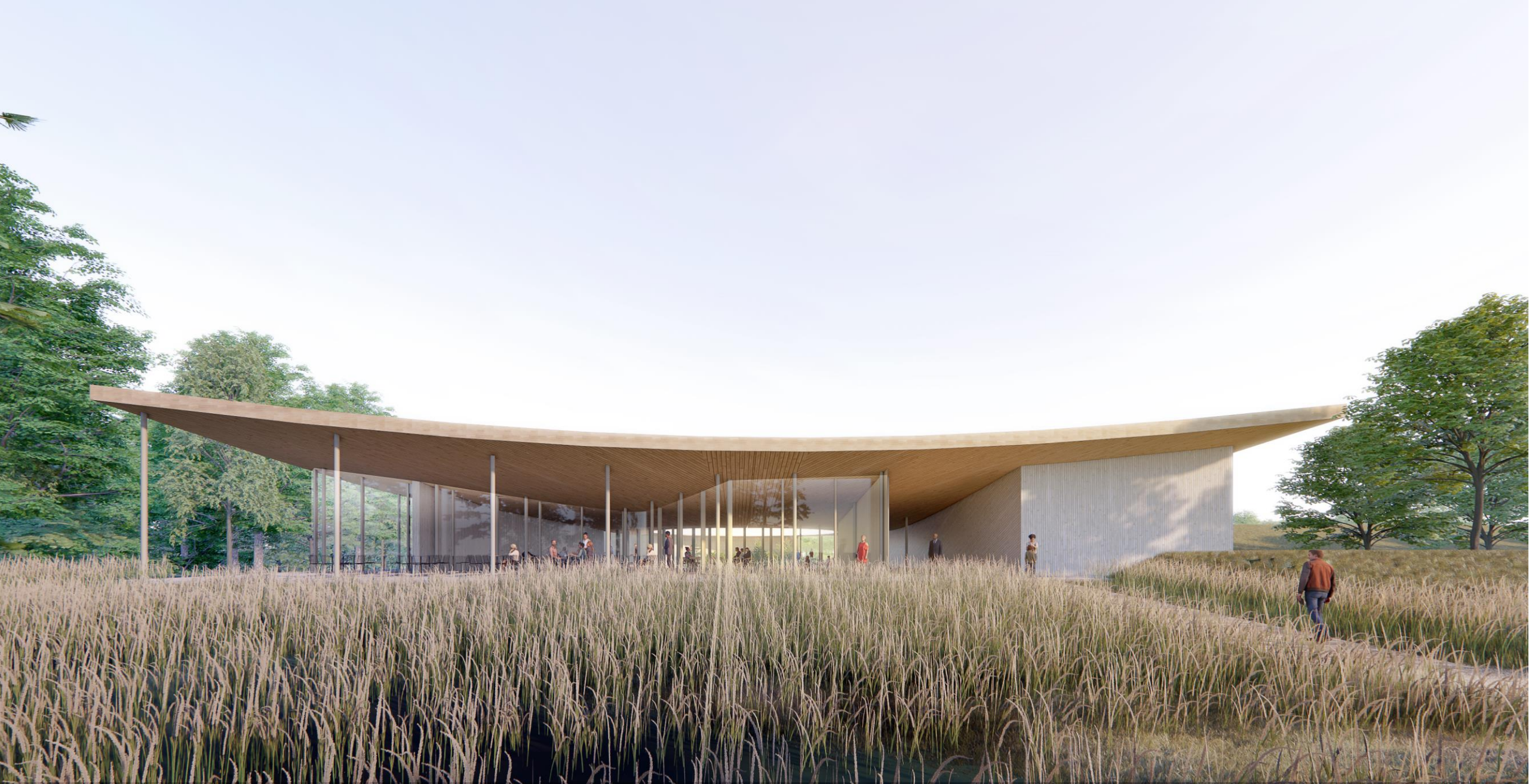
VIEW OF NORTH ENTRY
