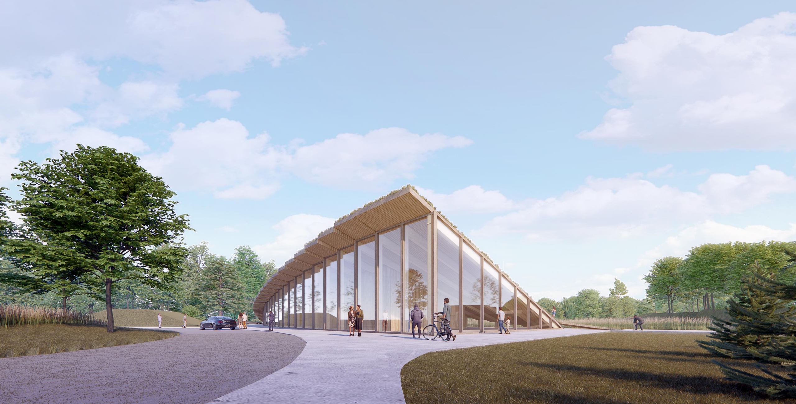
VIEW OF RECEPTION / MAIN SOUTH ENTRY
